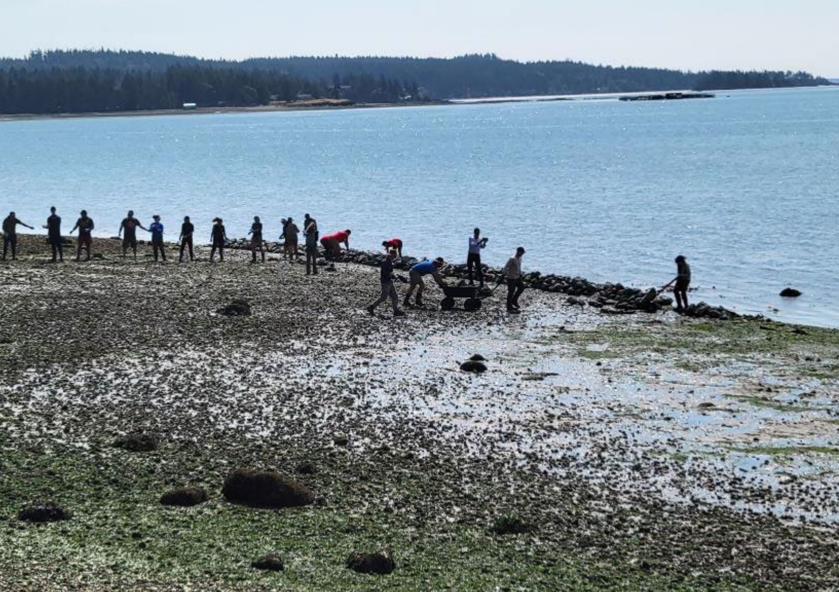
FIGURE 11: Pauquachin First Nation environmental stewards partnering with Swinomish tribal members at Kiket Island, lining up to pass stones for the creation of the first newly built clam garden in living memory, created by Swinomish for the first time in approximately 200 years, in August 2022. (Photo by Dr. Marco Hatch, Western Washington University professor and Samish Tribal Member.)
